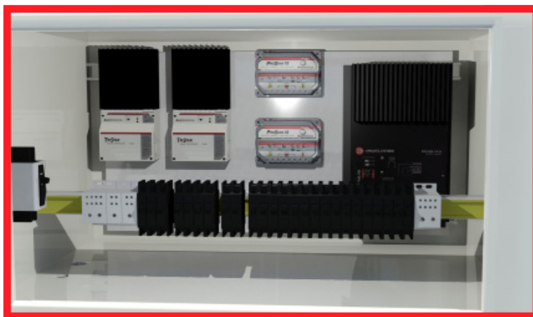
Mounting Tabs on Deadfront for DIN Breakers
