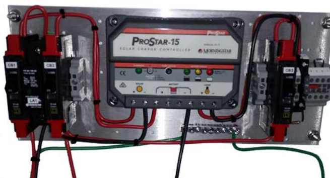
PRCP20 with a 15 amp ProStar charge controller
