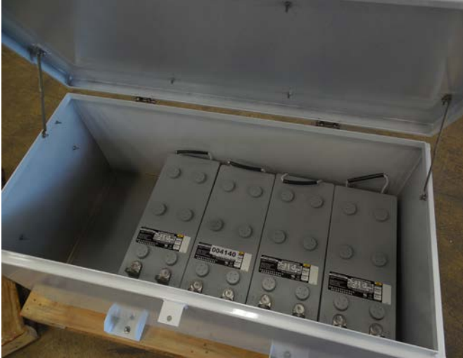
T-4X8D Enclosure with four 4D batteries
