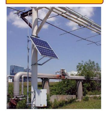
Smaller battery enclosures can be mounted on a pole or a wall. Usually up to 300-400 lbs, larger enclosures are placed on the ground, slab, or foundation. Practical limitations usually prevent too many batteries or too much weight from being installed on the pole or wall. Larger ground mount enclosures usually do not have any limits. Side of Pole enclosures offer easier access and maintenance to lighter-weight systems.
