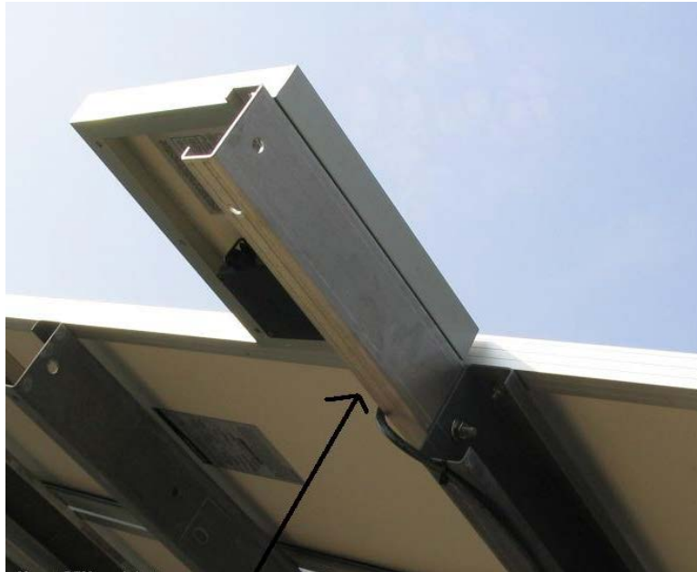
FIGURE 12: 10W PV MODULE FOR GENSET STARTER BATTERY
