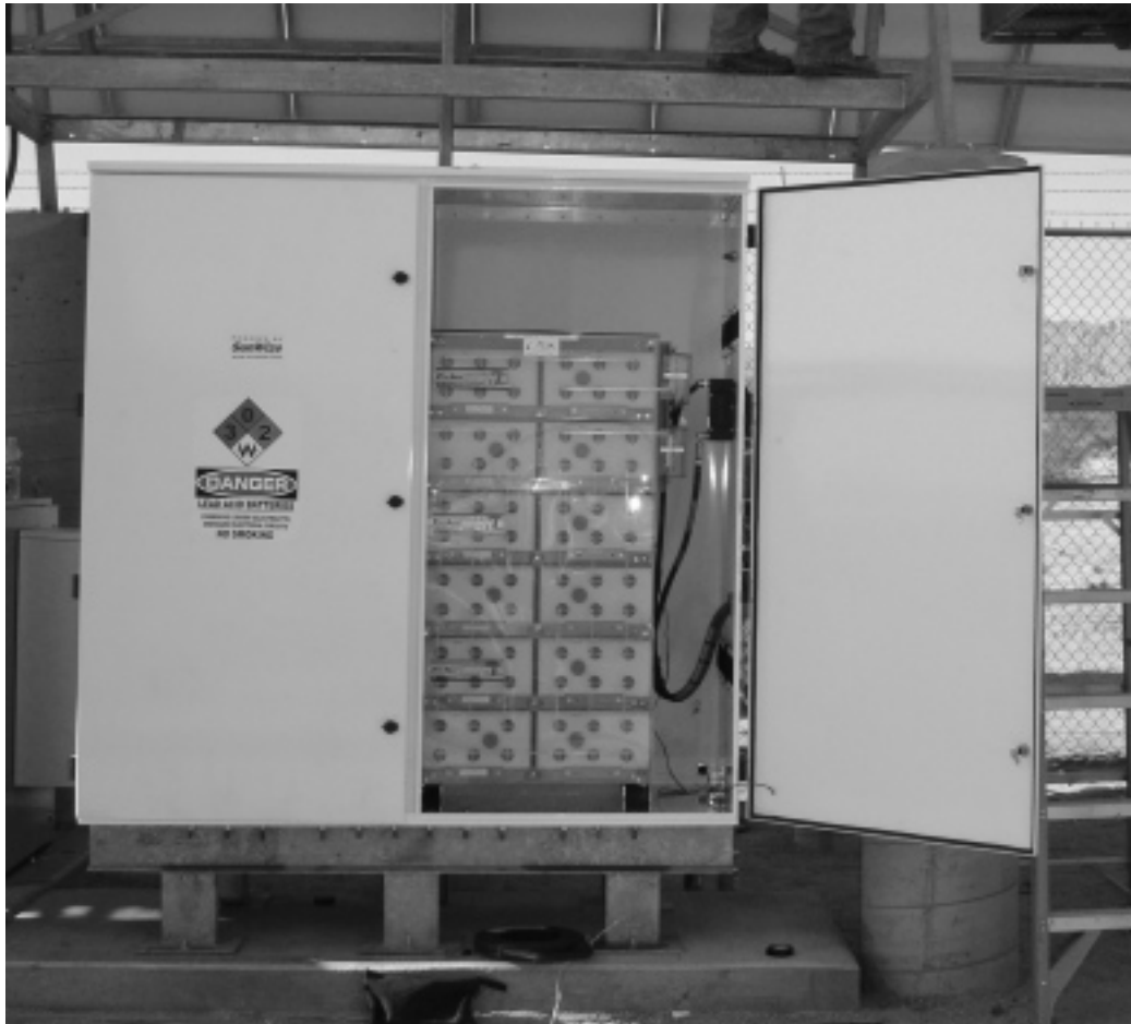
FIGURE 8A: PSF2-24 BATTERY ENCLOSURE
