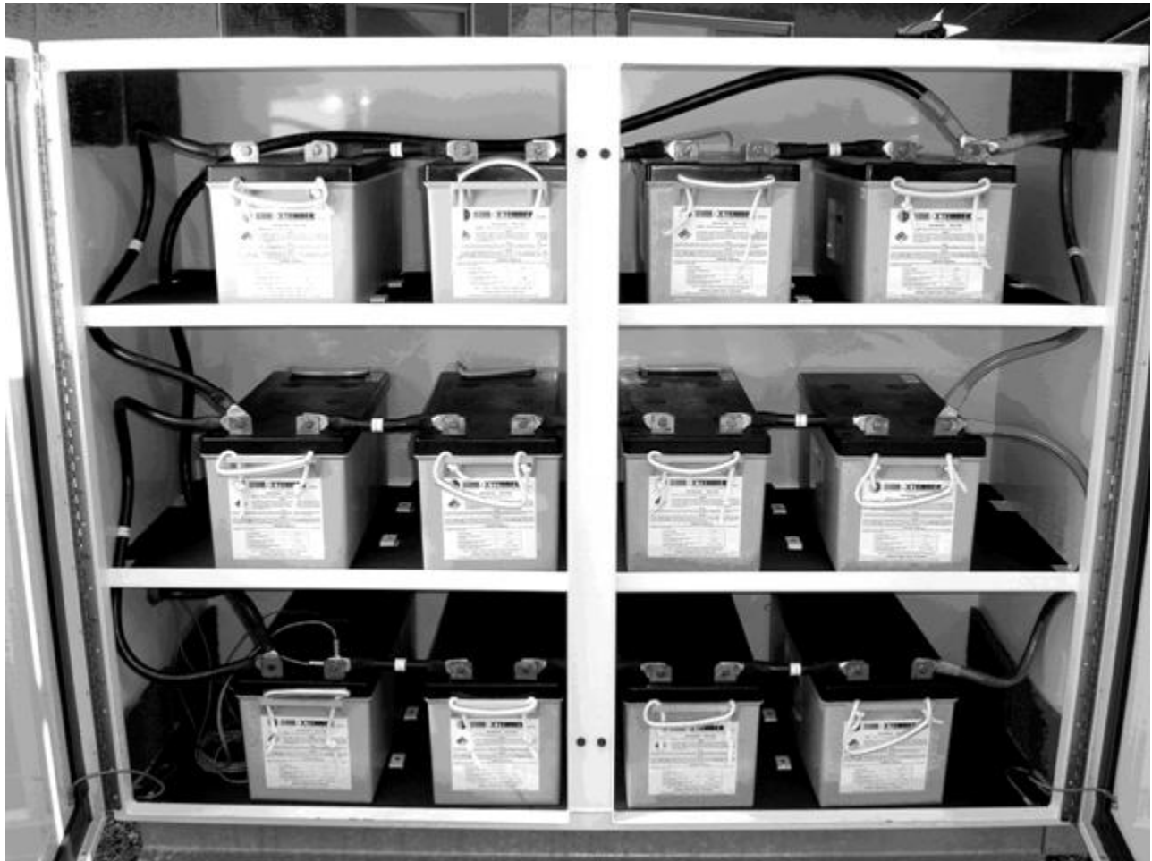
FIGURE 6A: PSF12-12 CONTROL/BATTERY ENCLOSURE
