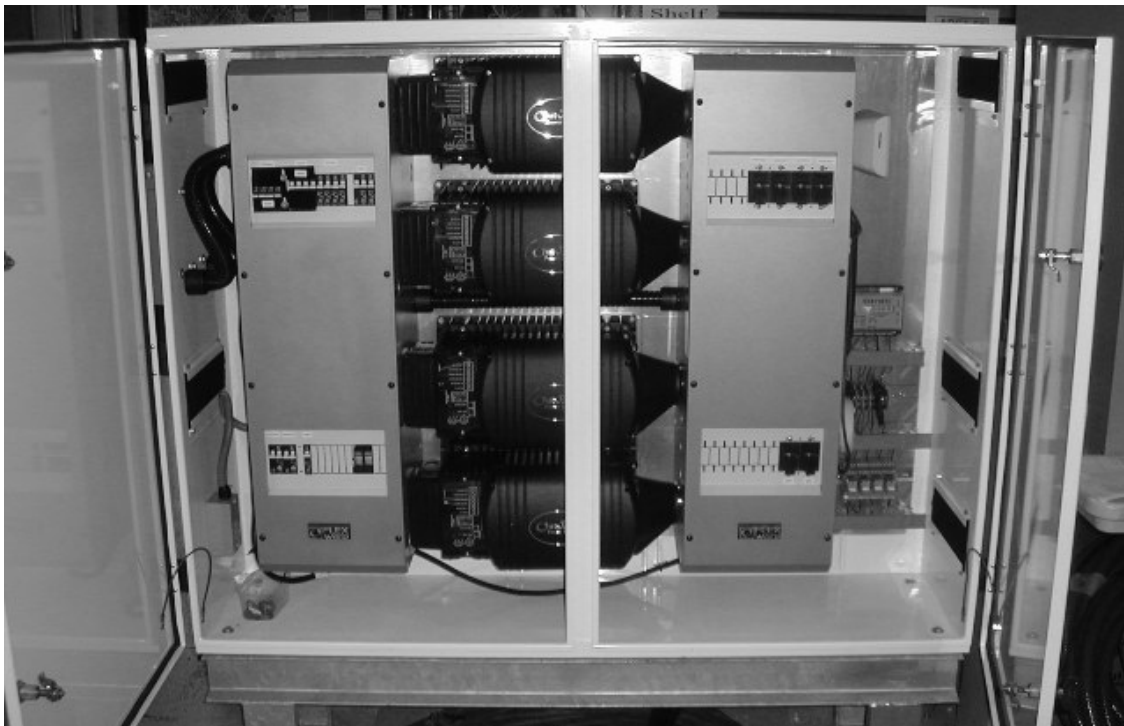
FIGURE 9A PSF-L CONTROL ENCLOSURE
