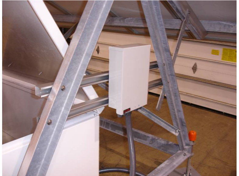
FIGURE11B: PV COMBINER S FRAME
