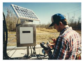
70°C. The SunKeeper is also certified for use in Class 1, Division 2 hazardous locations, making it an ideal controller for solar powered oil/gas applications.
