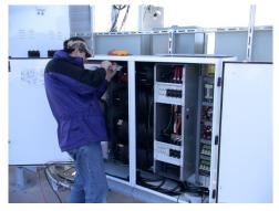
\*To protect batteries from becoming permanently damaged, systems will disconnect the load using a Low Voltage Disconnect "LVD" if battery energy ("State of Charge" or "SOC") drops below 20%!
