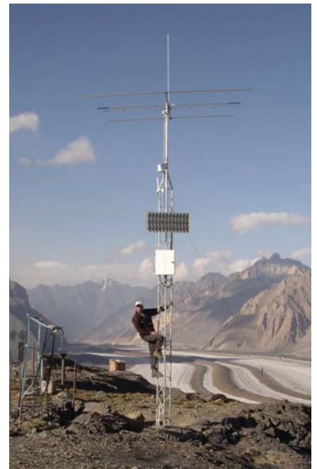
SunWize® Power Ready System in Tajikistan.
