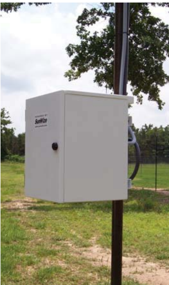
Corrosion resistant SunWize white powder-coated aluminum enclosure.
