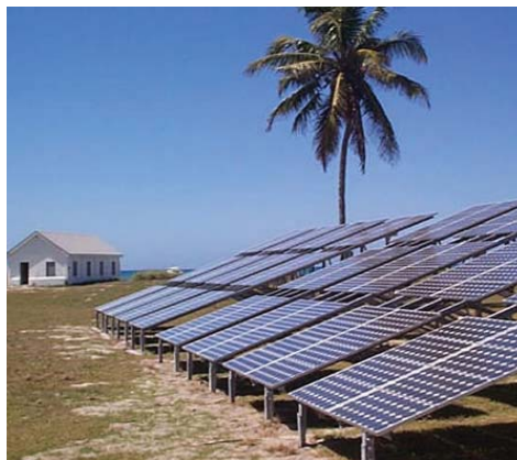
This Dry Tortugas National Park system has withstood hurricanes and years of salt water spray and continues to power employee housing and potable water production.
