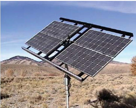
Incessantly subjected to extreme temperatures, this system provides power for a water pumping system in the US desert.
