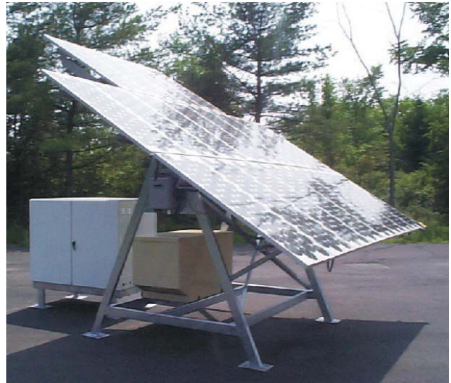
An 1800 watt solar /engine generator hybrid power system.
